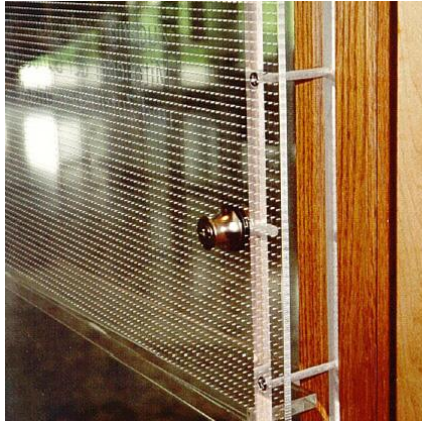
Microperforated polycarbonate panel absorber. Thickness 1 mm, hole diameter 0.65 mm
